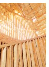
walls) to avoid hinge points that occur in platform-framed walls. The result is clean wall lines and a stable structure especially suited for large windows. As with PSL, a nail gun or other powered fastening tool makes installation easier.
