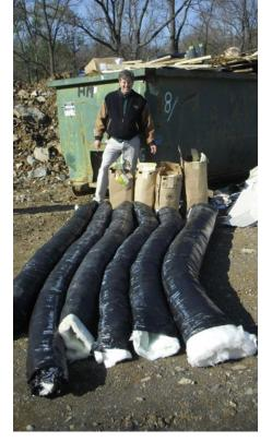
Here's a good example of waste: Scott Sedam pulled more than 80 feet of perfectly good insulated ductwork out of a jobsite dumpster. The "scrap" could have been used for short runs and "jumpers."
