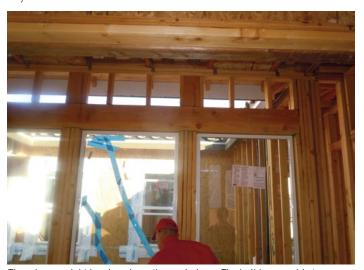
There is no weight bearing above these windows. The builder was able to remove 12 king studs and 14 cripples across the entire span, saving more than 130 feet of lumber with no detriment to the house.
